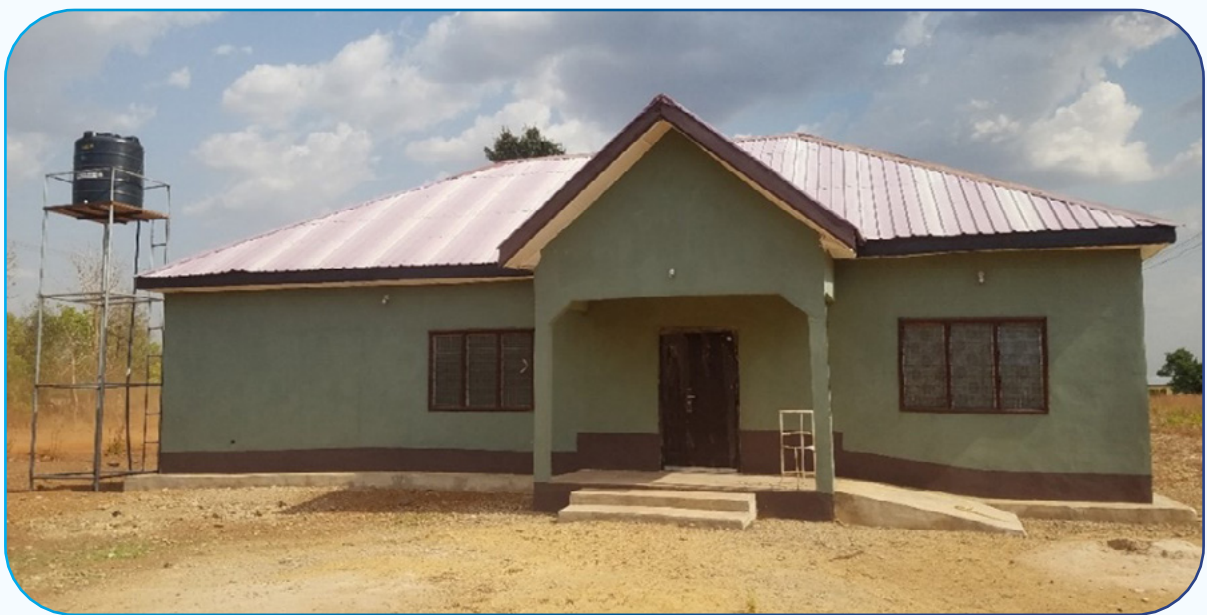
P4H empowered CHMC advocacy resulted in the building of a New CHPS Compound for resident of northern region town of Kotingli by the Tamale South Legislator
