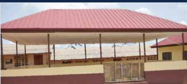
Picture: The cafeteria section of the new school.
